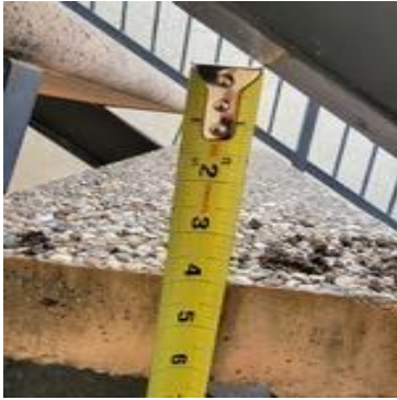
Picture 279: Railing of stairway
