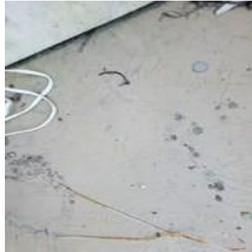
Picture 92: Surface of stairway
