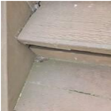
Picture 98: Surface of stairway
