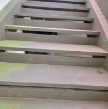
Picture 94: Surface of stairway
