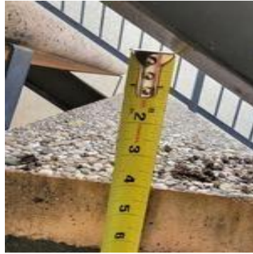
Picture 280: Railing of stairway
