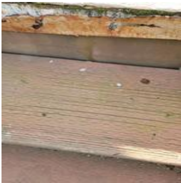
Picture 103: Surface of stairway
