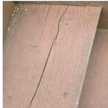
Picture 100: Surface of stairway
