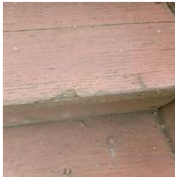
Picture 104: Surface of stairway
