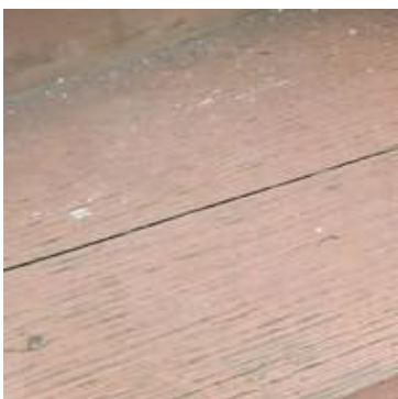
Picture 101: Surface of stairway
