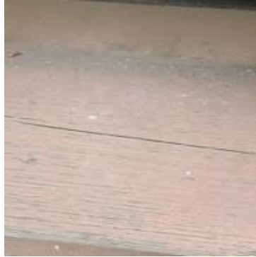
Picture 96: Surface of stairway
