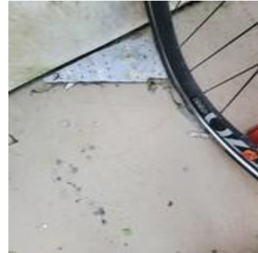
Picture 93: Surface of stairway
