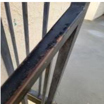
Picture 281: Railing of stairway
