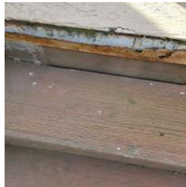
Picture 105: Surface of stairway
