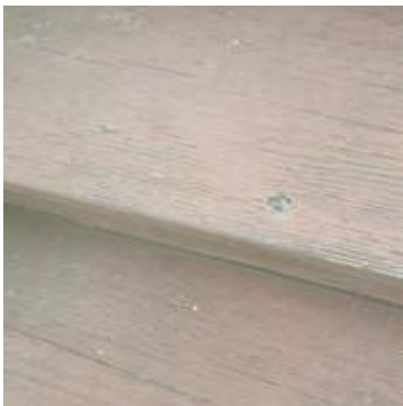
Picture 106: Surface of stairway
