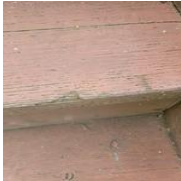
Picture 99: Surface of stairway
