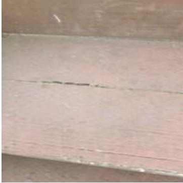
Picture 95: Surface of stairway
