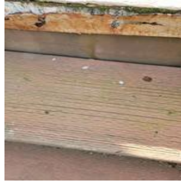
Picture 97: Surface of stairway
