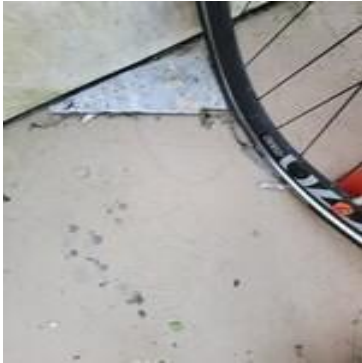
Picture 91: Surface of stairway
