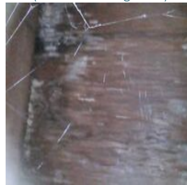
Picture 360 ( Defect Code: 137 )
