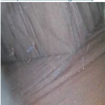
Picture 486 ( Defect Code: 147 )
